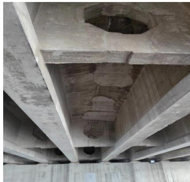
Considering that Jiangbei Bridge has been in service for a long period, and in order to enhance the durability of the prestressed T-beam concrete and extend its service life, it was decided to use the XYPEX Concentrate crystalline slurry coating system for surface rehabilitation and strengthening.
